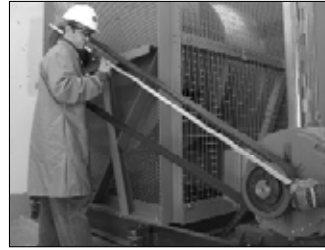
Using a straight edge to check alignment
