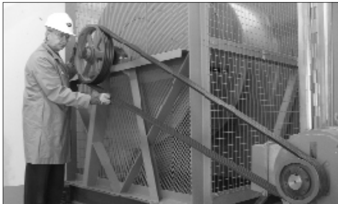
Begin by inspecting the belt
